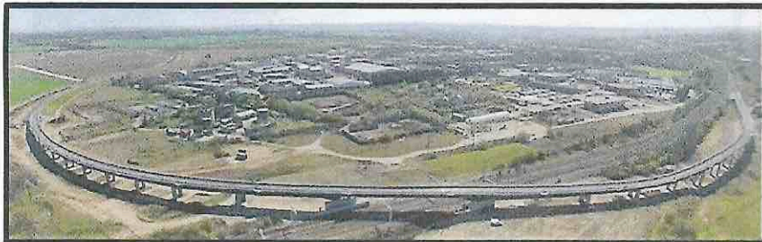
This is a panoramic view of the complete structure.
