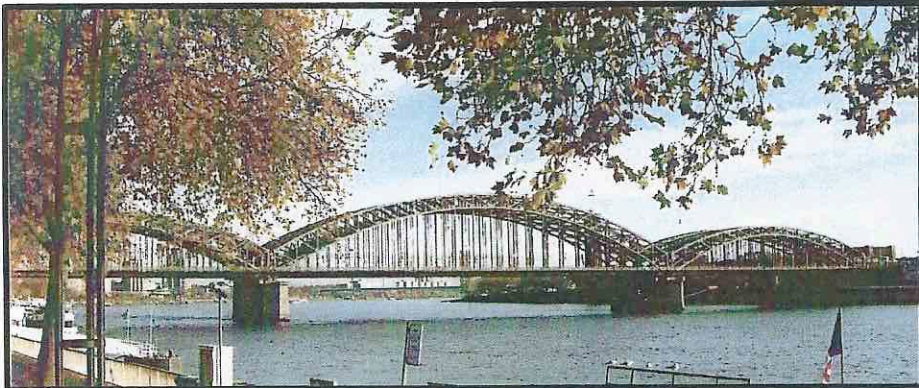
Hohenzollern Bridge over the Rhine that has 6 railway tracks on it and is (usually) very busy.
