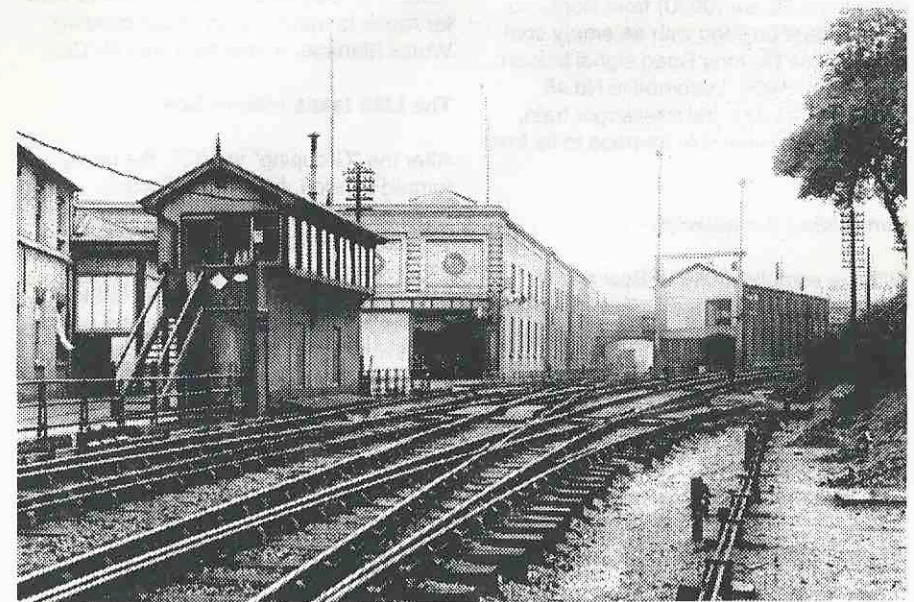
Bow Works, view towards Poplar, link to LT&S on right
