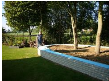
Track laying begins, we put a layer of underfloor heating insulation board all-round the top of the wall. I painted it grey using some garage floor paint that we had, this turns it from the odd blue colour to a more acceptable grey. Tim Breeze is the contractor that is laying the track as this was a job I had not undertaken before and the track is not cheap.
