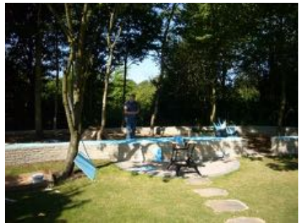
Track laying begins, we put a layer of underfloor heating insulation board all-round the top of the wall. I painted it grey using some garage floor paint that we had, this turns it from the odd blue colour to a more acceptable grey. Tim Breeze is the contractor that is laying the track as this was a job I had not undertaken before and the track is not cheap.
