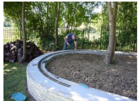
Track laying begins, we put a layer of underfloor heating insulation board all-round the top of the wall. I painted it grey using some garage floor paint that we had, this turns it from the odd blue colour to a more acceptable grey. Tim Breeze is the contractor that is laying the track as this was a job I had not undertaken before and the track is not cheap.
