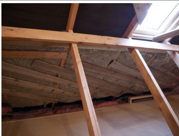
Picture 13 Rockwall and battens on front lower wall
