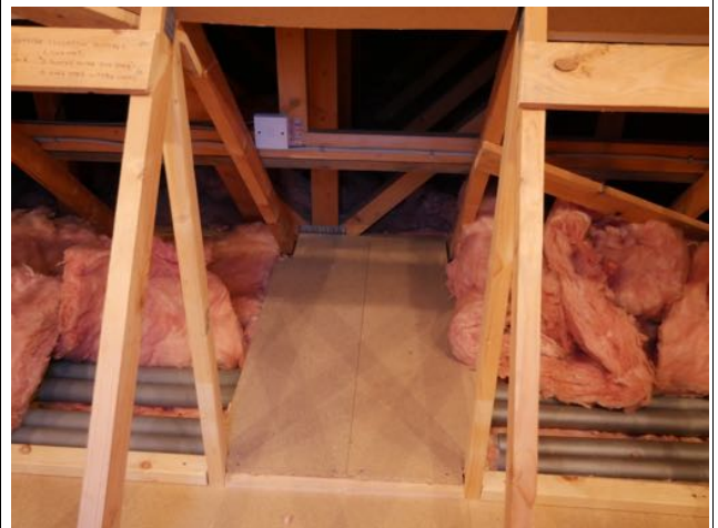
Picture 8 Kitchen loft access area and uprights. Note diverted central heating pipes, "path" into loft and insulation
