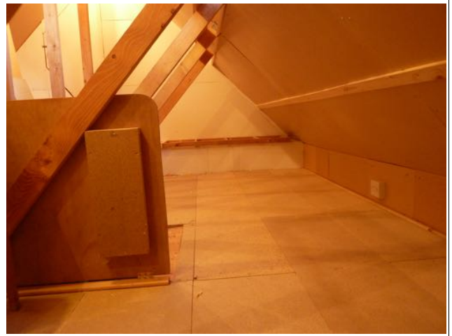
Picture 16 Under the front eaves, showing the loft safety hinged floor piece.
