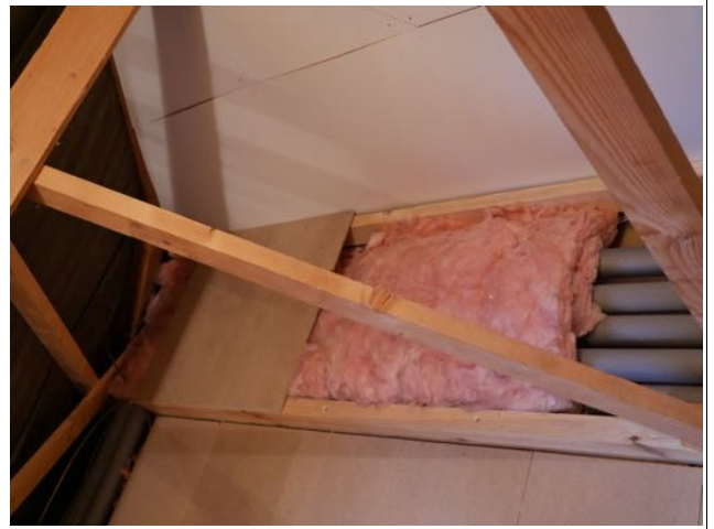
Picture 10 Pipes being covered with insulation and slightly higher floor going in.
