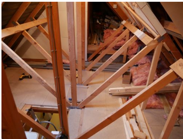
Picture 7 Main floor laid. Note uprights on R/H side, some insulation and part of sandwich wall in.
