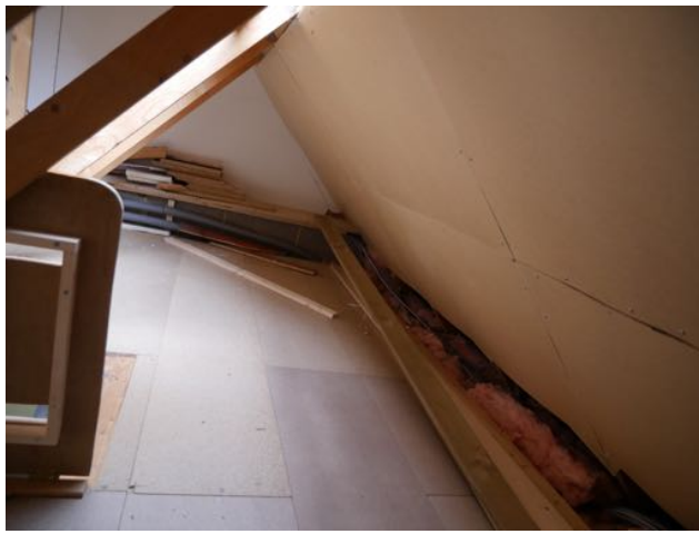
Picture 15 Hardboard covering battens right down to within 1 foot of eaves, leaving access to a cable run along the front.
