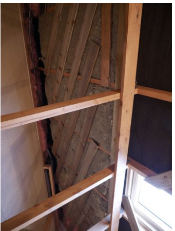
Picture 11 One end sandwich wall with door thro' to ordinary loft area.
