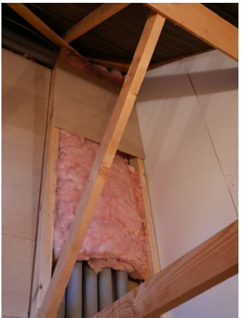
Picture 10 Pipes being covered with insulation and slightly higher floor going in.
