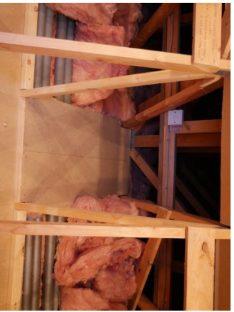
Picture 8 Kitchen loft access area and uprights. Note diverted central heating pipes, “path” into loft and insulation
