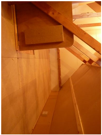
Picture 16 Under the front eaves, showing the loft safety hinged floor piece.
