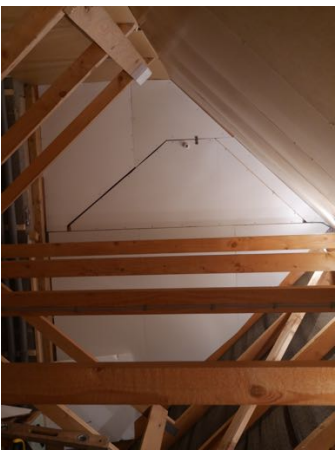
Picture 9 Same area, Different angle with insulation and hardboard going in.
