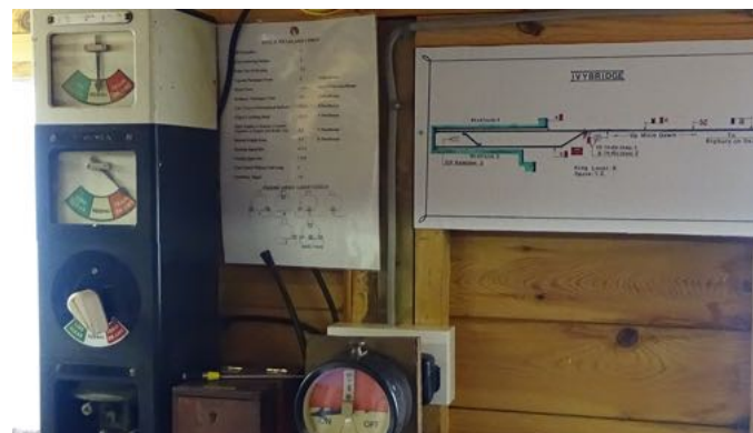
Ivybridge signalling diagram and block shelf.
