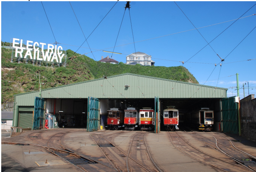
The Manx Electric Railway running shed at Derby Castle, Douglas. The friendly member of staff gave me a personal conducted tour, the maintenance sheds stand off to the left.
